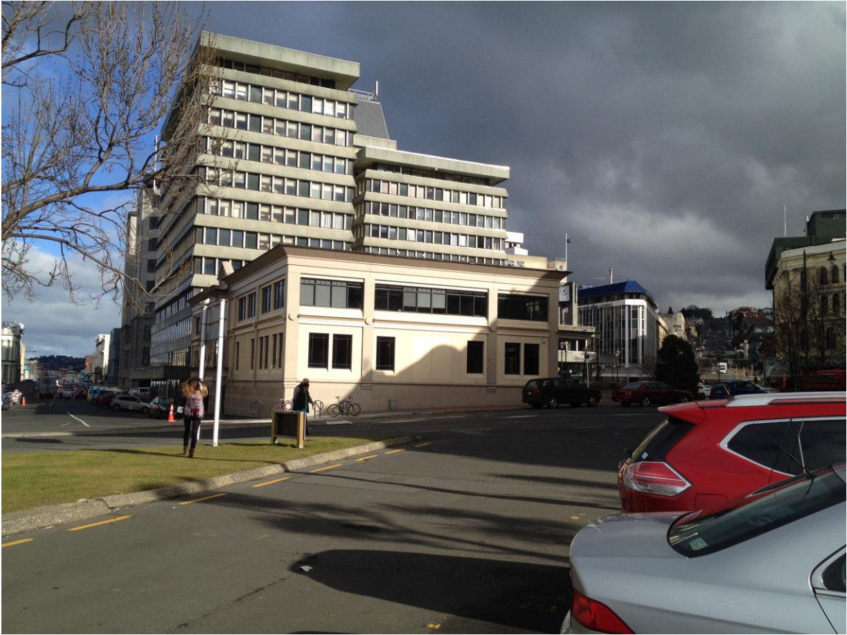
Figure 1 - Exterior View of Northern Wall viewed from Rattray Street
