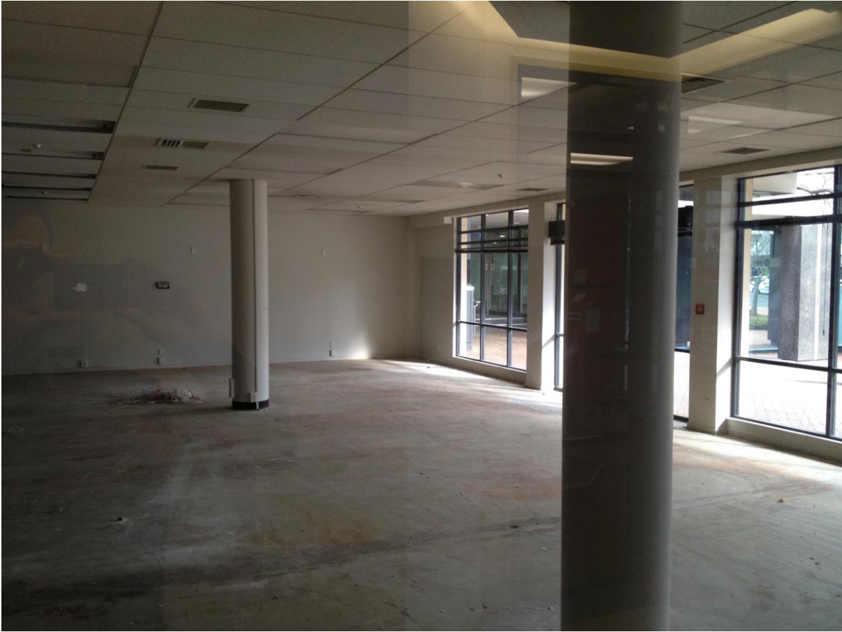
Figure 3 – Interior View of Ground Floor office space looking south-west
